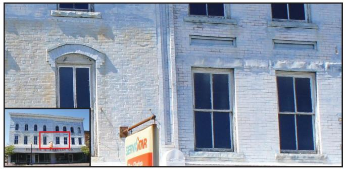
Fig. 16 - Detail of façade showing common bond on south side (at left) and running bond on north side (at right) (Detail location in relation to rest of the façade shown at bottom left)
